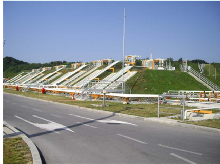
Cylindrical lying tanks covered with a layer of earth
