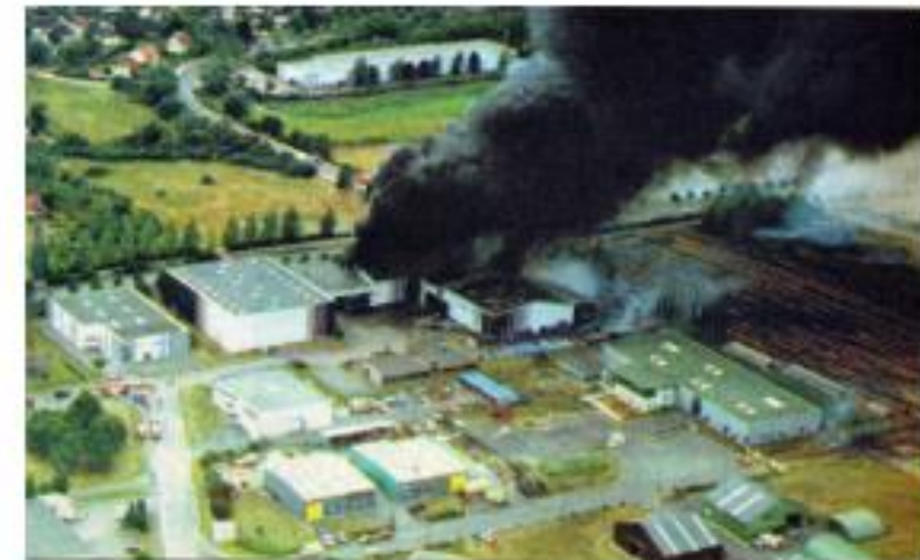
Figure 1. Explosion and fire at agrochemicals warehouse, 6/8/1996
