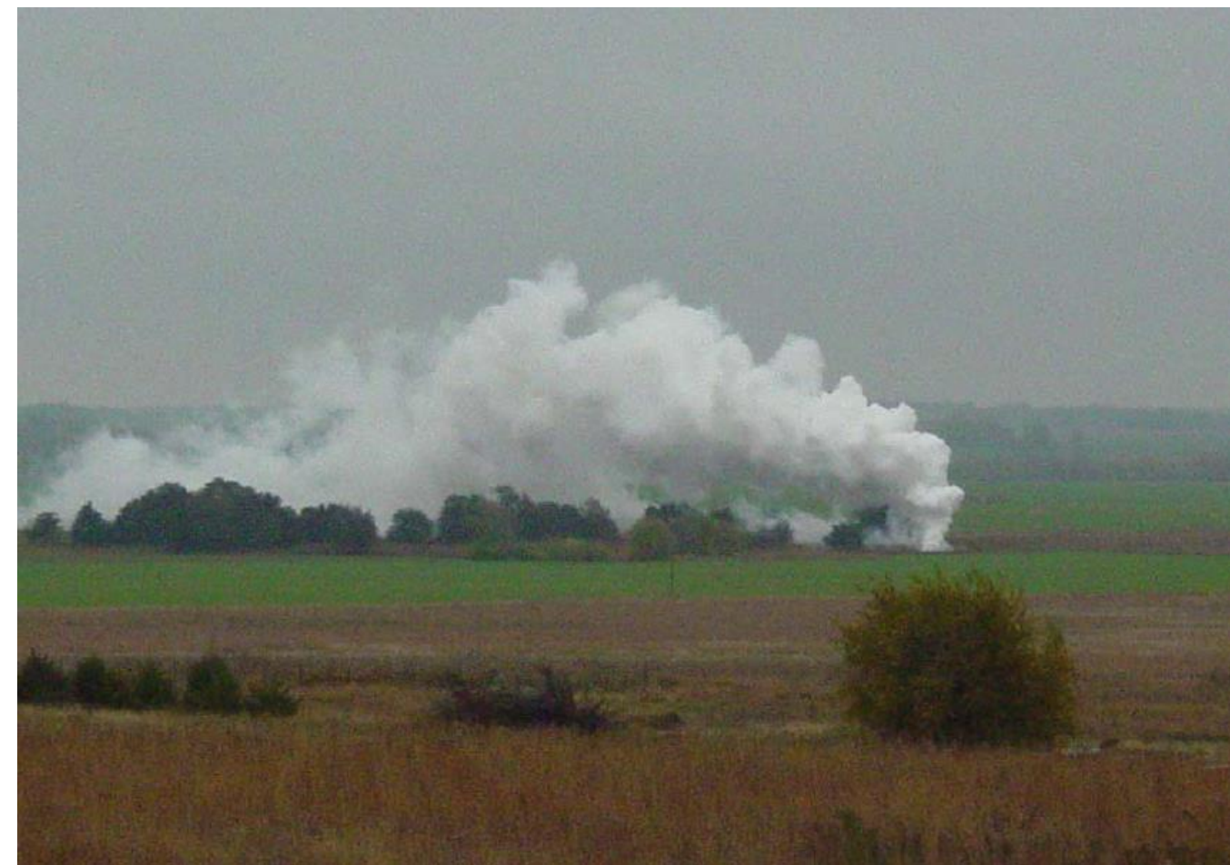
Ammonia pipeline release, Kingman, Kansas (2004)
