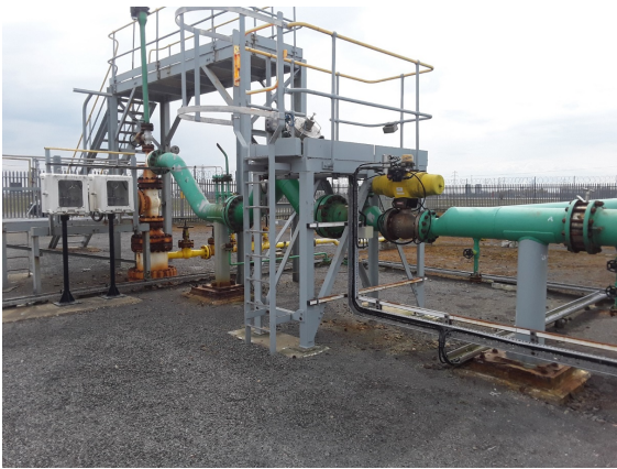
Cavern storage wellhead. Courtesy SABIC
