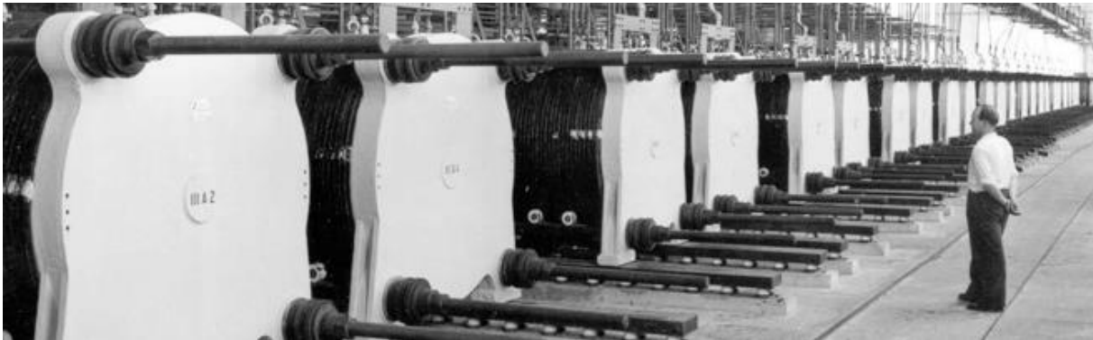
135 MW hydro-power electrolysis-based hydrogen production in Glomfjord, Norway 1953-1991
