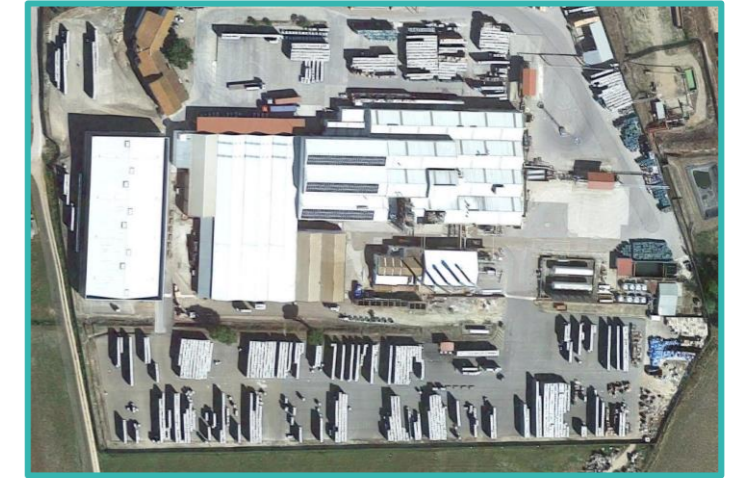
LNG storage (UAG) at a tomato processing plant
