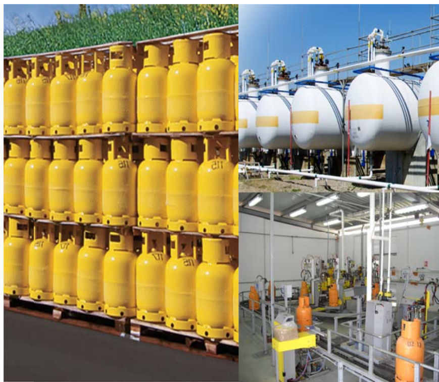
Figure 3 Various types of LPG installations
