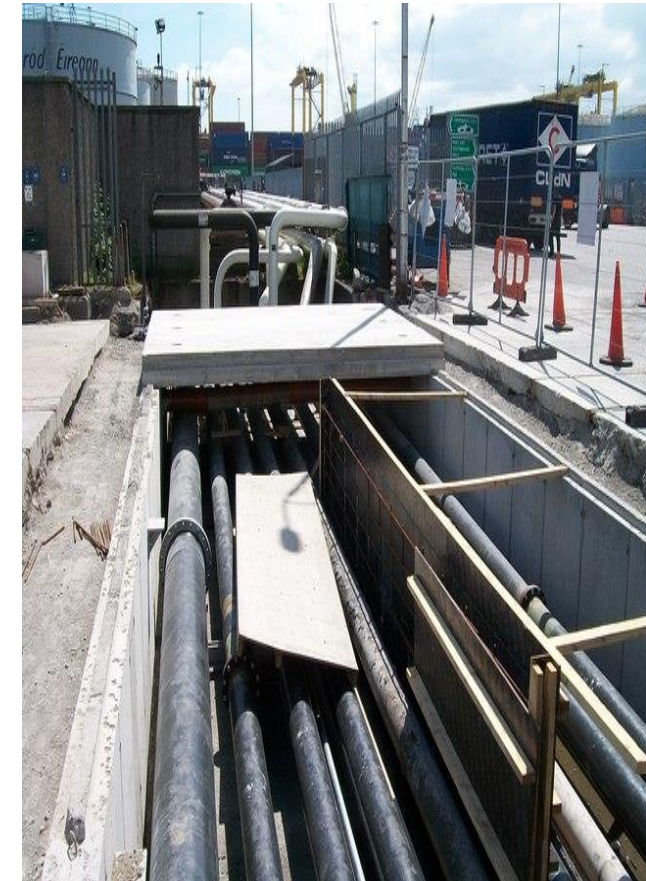
Oil pipelines exposed for maintenance (Photo credit: Eric Jones)
