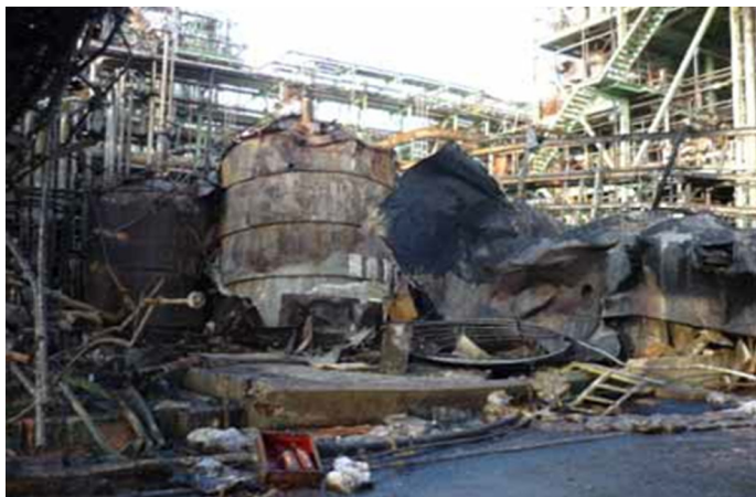
Figure 5: The acrylic acid intermediate tank after the explosion (Source: Investigation report)
