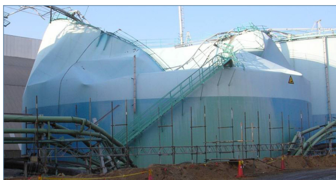
Figures 1 and 2: The damaged tank and underground pipeline (Source: Swedish Investigation Board report).
