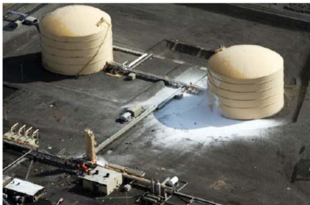
Figure 2. Aerial view taken shortly after the failure. Fires still burning. Perlite insulation leakage from the penetrated outer LNG-1 storage tank. Control room lower left. (PHMSA, 2016)
