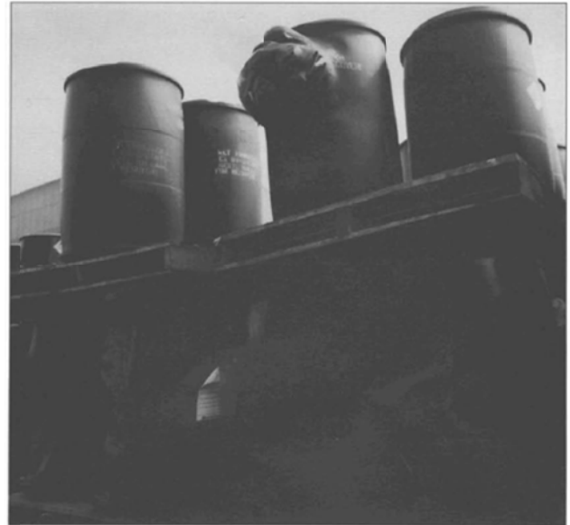
Figure 3: Plastic drums on the fire block flammable liquid storage area showing heat radiation damage and effects of pressurisation. (HSE, 1992)
