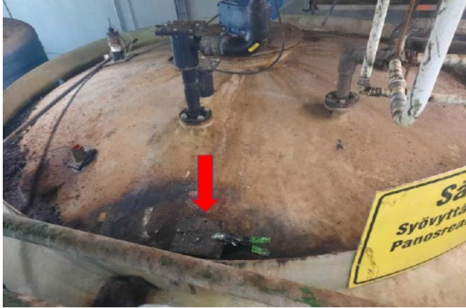
Figure 2. Sampling area of toxic gas release on the top of the waste treatment reactor (Source: Tukes, 2022, Chemical reaction at a waste recycling plant_2022.pdf )
