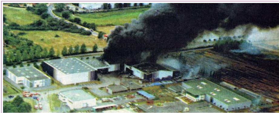
Figure 1. Explosion and fire at agrochemicals warehouse, 6/8/1996 (Source: https://www.estrepublicain.fr/ )
