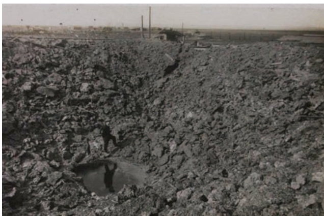
Figure 2 – Crater created by explosion of building 217 (note man in centre)
