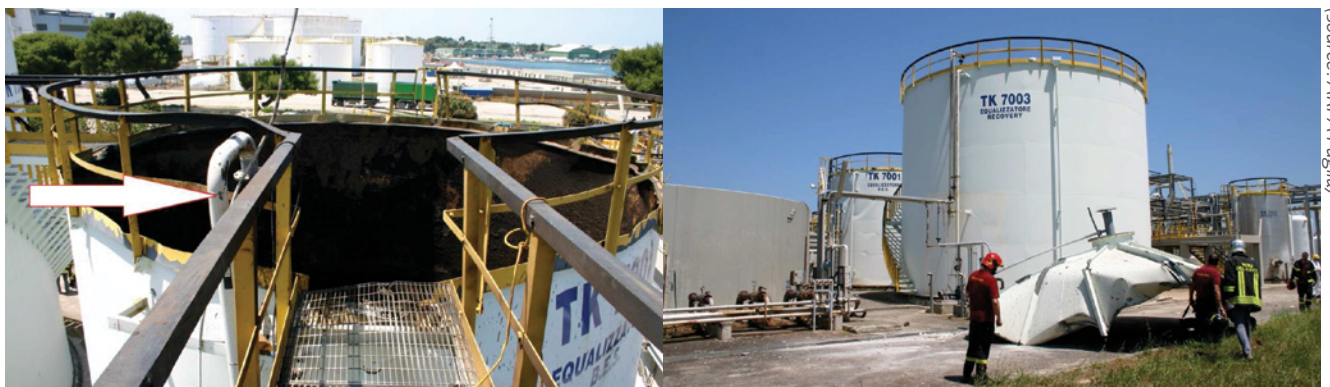
Figure 3 – Pulled-off sparger line on the TKX viewed from the walkway and the projected roof at the foot of the TKX
