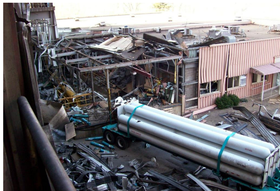
A fatal hydrogen explosion occurred while a tube trailer (right) filled onsite hydrogen storage cylinders (yellow tanks, left).
