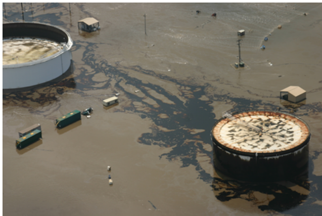
Figure 1. Oil slick formed after flood damage to storage tanks in Coffeyville, USA, 2007 (Photo credit: Kansas Civil Air Patrol)
