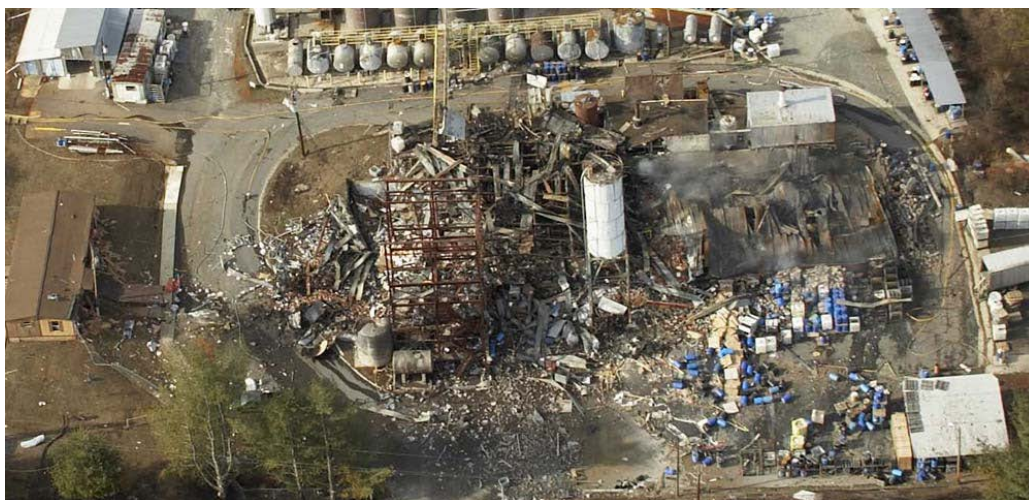
Figure 2: Synthron facility after the explosion (CSB report 6 )
