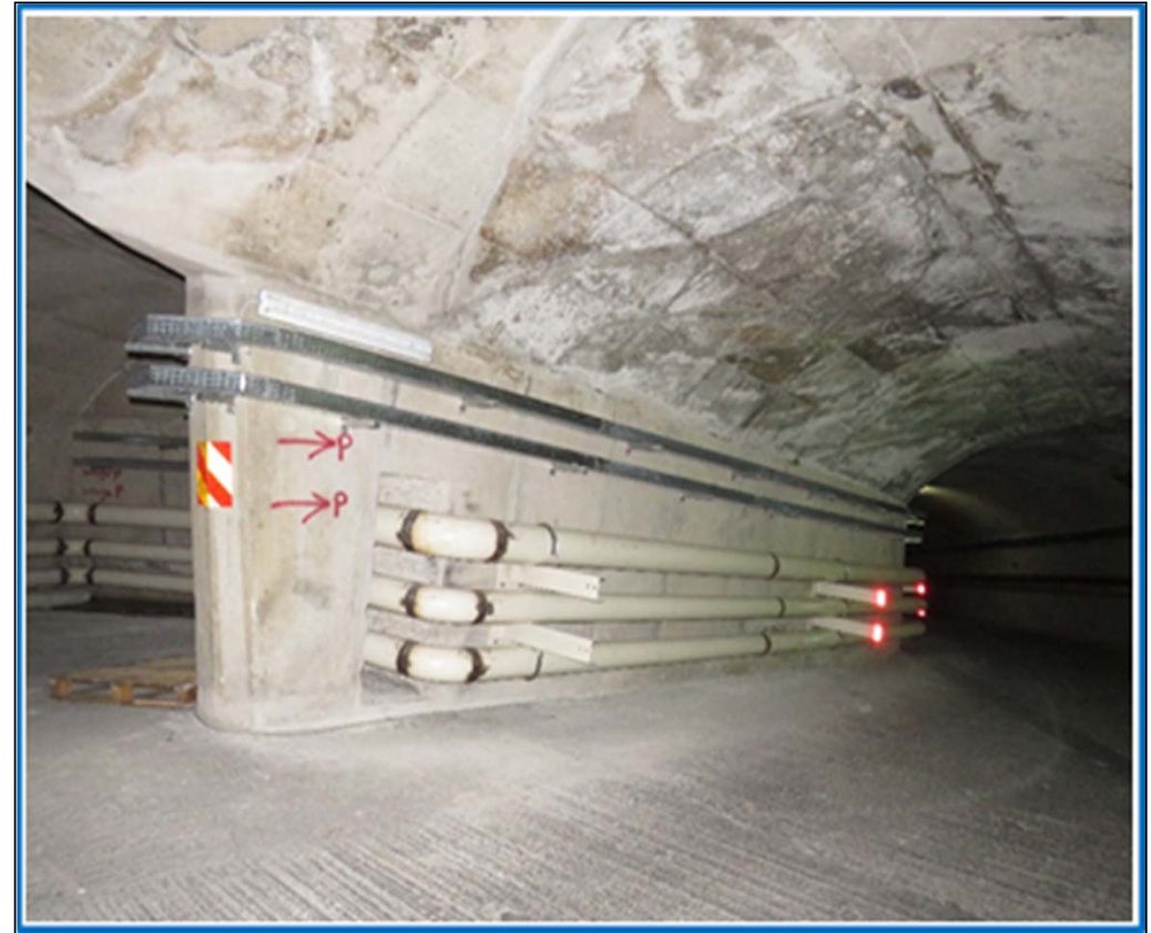
New Pipeline Network
