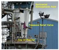
Figure 1. Reactor with a pressure relief system (U.S. Chemical Safety Board, 2018)
