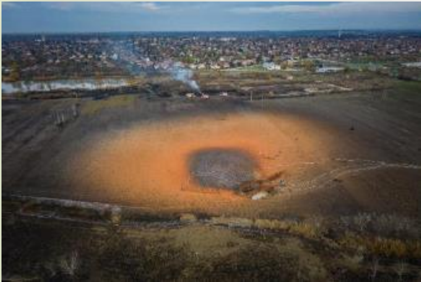
November 2019. CNG explosion 64 bar DN800 1,7 million m 3 methane
