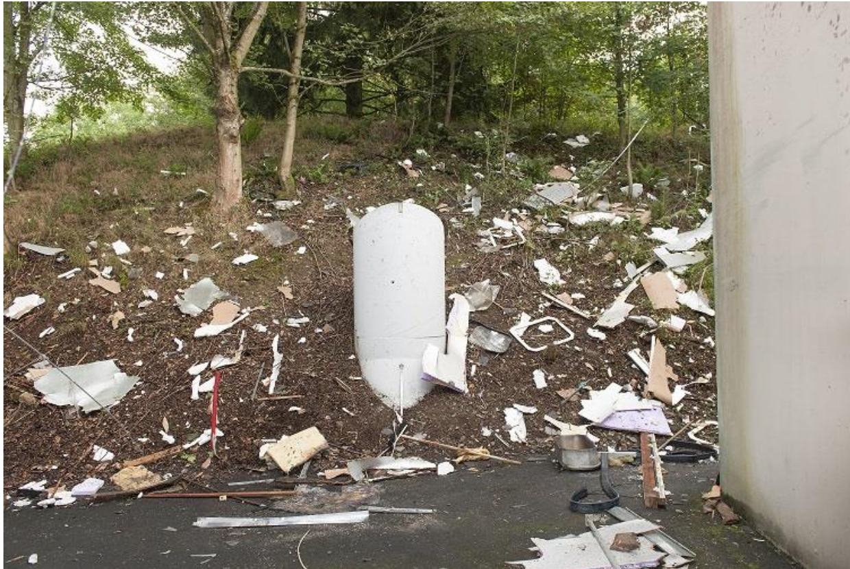
exterior view from box to wall
