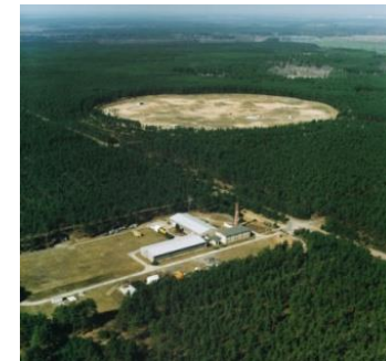
BAM Test-site Technical Safety in Baruth/Mark
