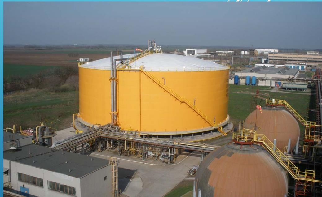
AMMONIA STORAGE DEPOTS - LP- tank, 103.8 kPa (2.5 kPa, - 33 °C, 22300 m<sup>3</sup> - 15000 t NH<sub>3</sub>, h = 15 m, d = 43.5 m), ALDUR 50D, 1970
