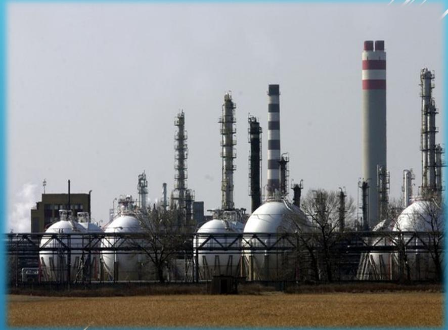
LPG STORAGE DEPOTS - spherical LPG storage tanks, 1000 m<sup>3</sup>,
