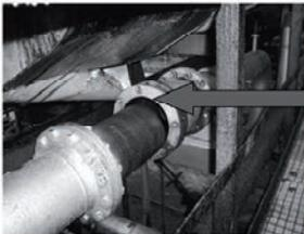
defect axial expansion joint (axial compensator)
